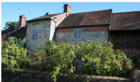
Mill House, The Dene
